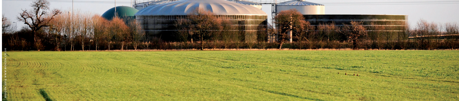
The Westwood AD plant in Northamptonshire, UK, processes 65 000 tons of food waste per year to produce power injected into the grid.
