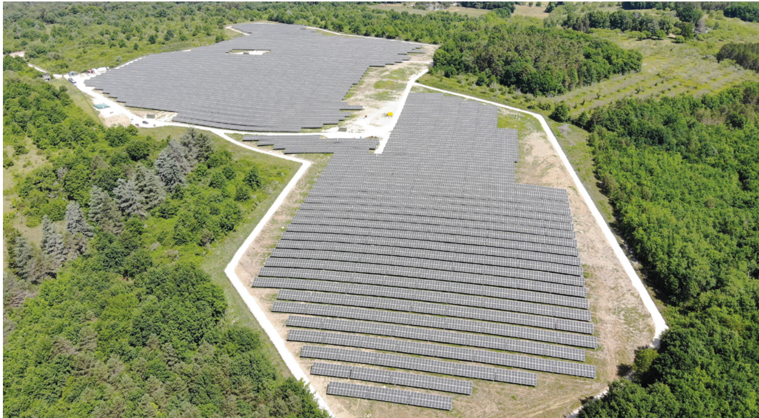
The Eyliac solar power plant, located in Gironde, has been supplying Bonduelle with 13 GWh of solar electricity annually since January 2024.
